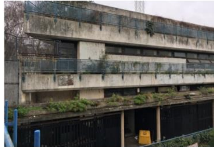
1. View of TRA Hall/Community Centre looking north from link bridge
