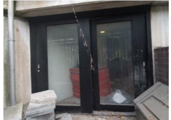
2. View of Existing Doors from Bin Store.
