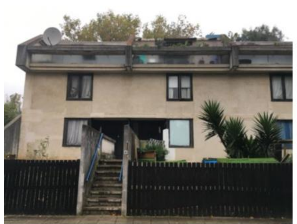
Block C from Boundary road (South elevation)
