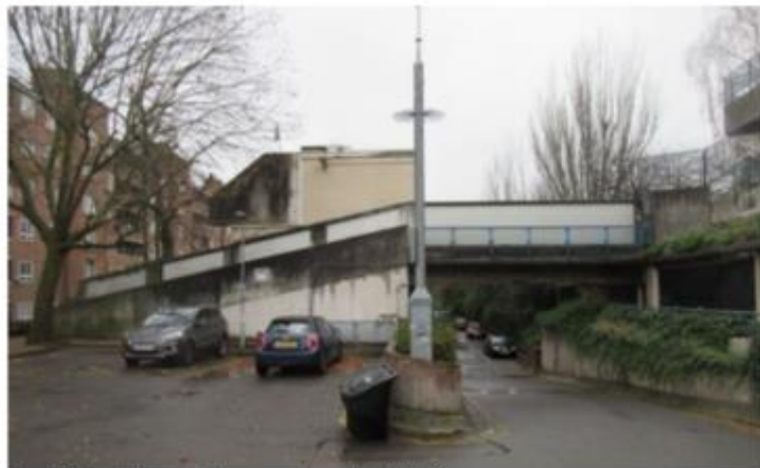
View 1: Bridge link between the community centre & block C.
