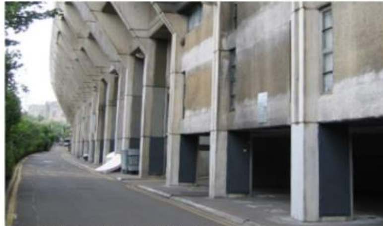
1. Existing Block A ground condition - North Elevation
