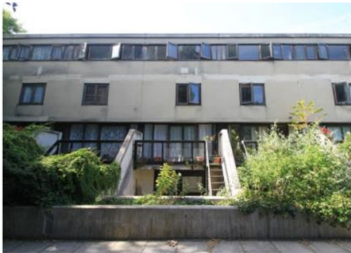
Block B South Elevation, seen from Langtry Walk
