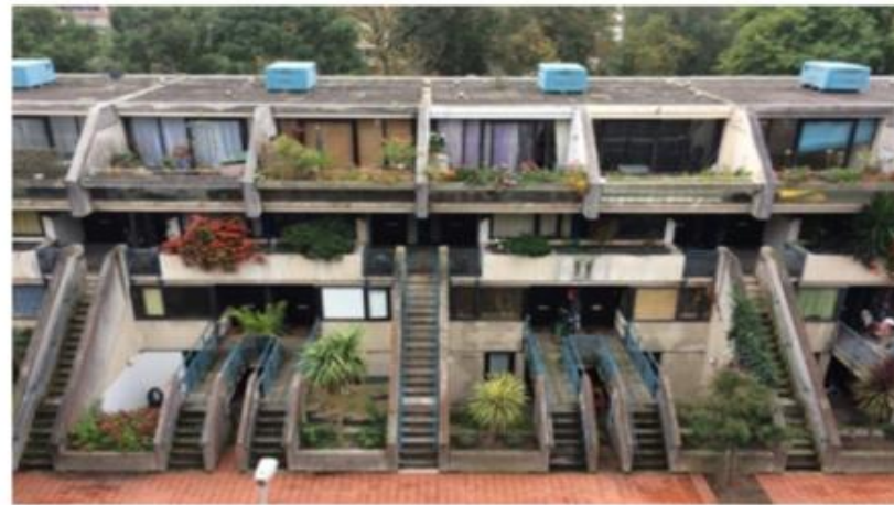
View of block B roof from Block A - Existing
