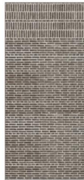
Top brick frieze: Alternating one row of headers, two rows of soldier courses
