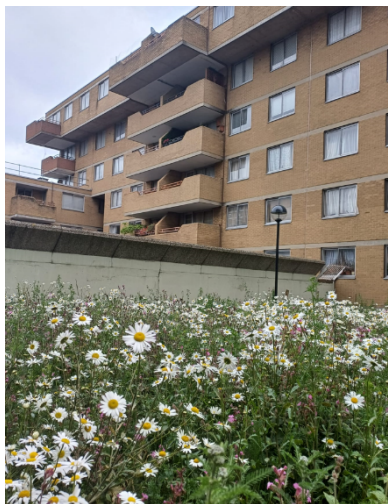
Meadow on the roof at Gamages
