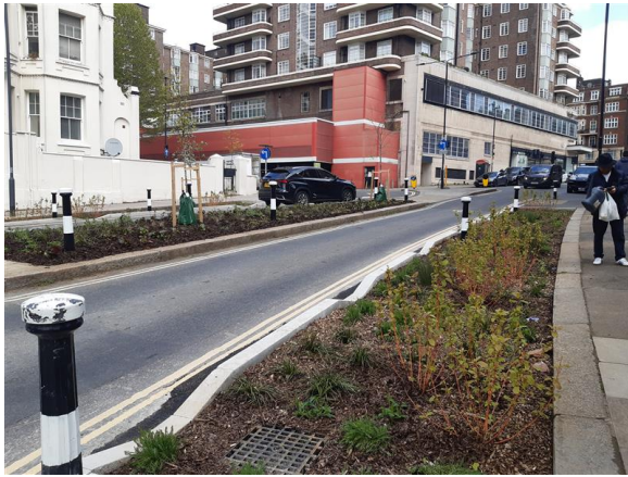
Goldhurst Terrace rain gardens works
