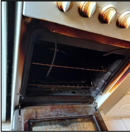
Communal cooker with defective heat seal and scorched controls.
