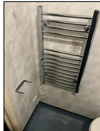
New heated towel rail installed
