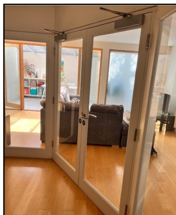
3 Inner rooms required fire protection via the installation of this partition.
