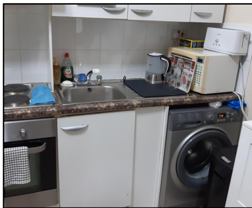
Communal kitchen with insufficient worktop, plug sockets and poor layout
