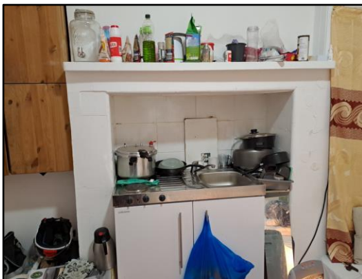
"Kitchenette" with inadequate space, worktop provision, food storage, power sockets and general layout.
