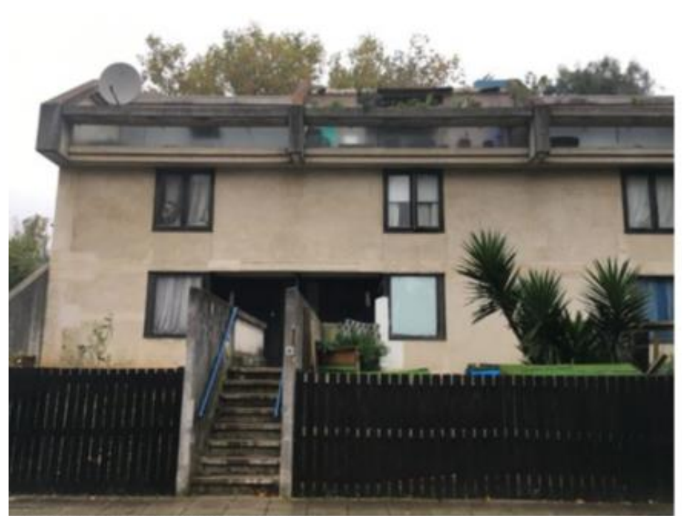
Block C from Boundary road (South elevation)
