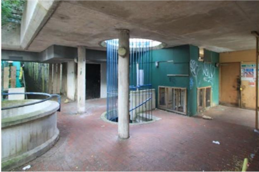
North of boiler room - Existing temporary timber hoarding on site
