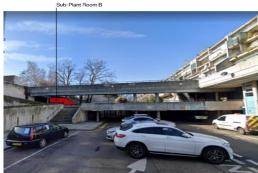
View from level 02 of car park entrance with proposed Sub-Plant Room B highlighted
