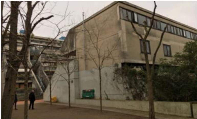
Block B West gable elevation - existing
