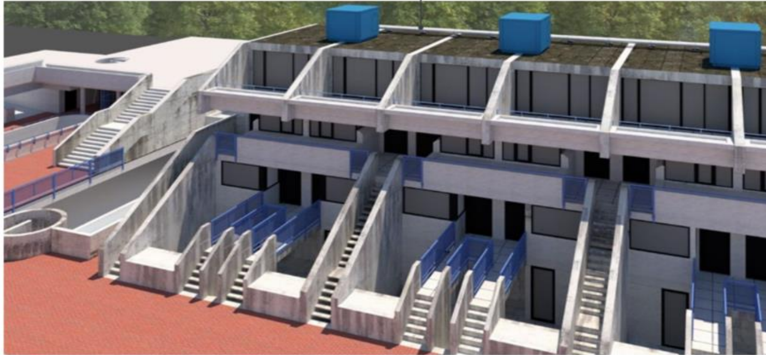
View of block B roof from Block A - Proposed
