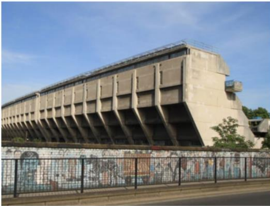
Block A north facade from Abbey road
