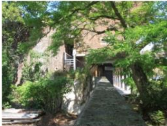
2. Loudoun Road Block West elevation. Proposed heating pipes externally fixed to wall at ground floor level behind existing external staircase.
