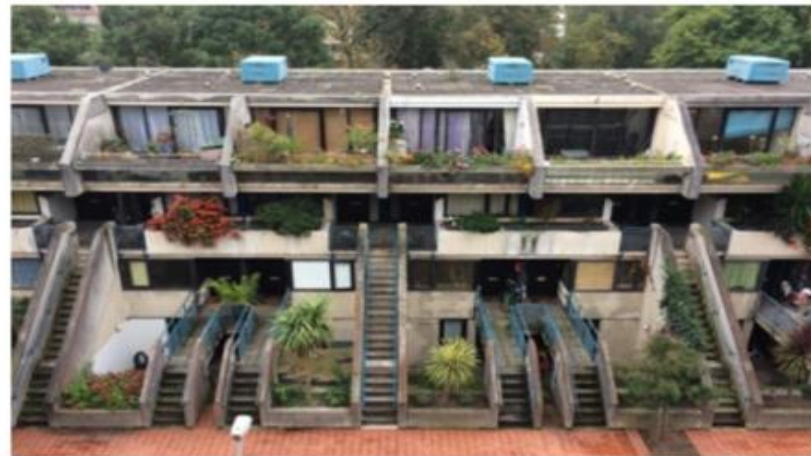
View of block B roof from Block A - Existing
