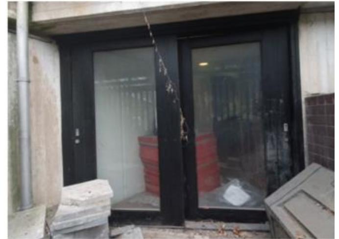
2. View of Existing Doors from Bin Store.
