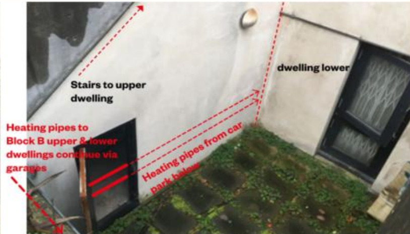
Block B, Dwelling type B3 external ground floor terrace (Rowley way)
