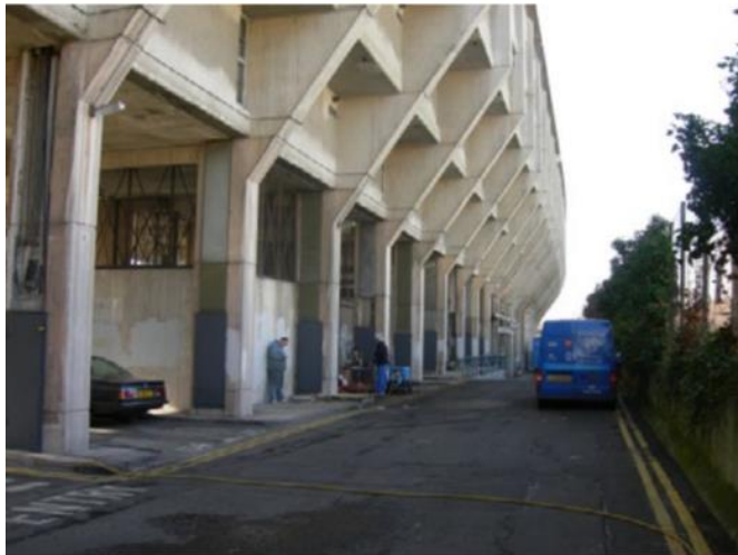
Block A looking west along service road to north
