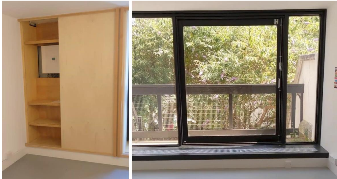
Figure 5 (above): New HUI (left) and refurbished windows (right) in a pilot flat
