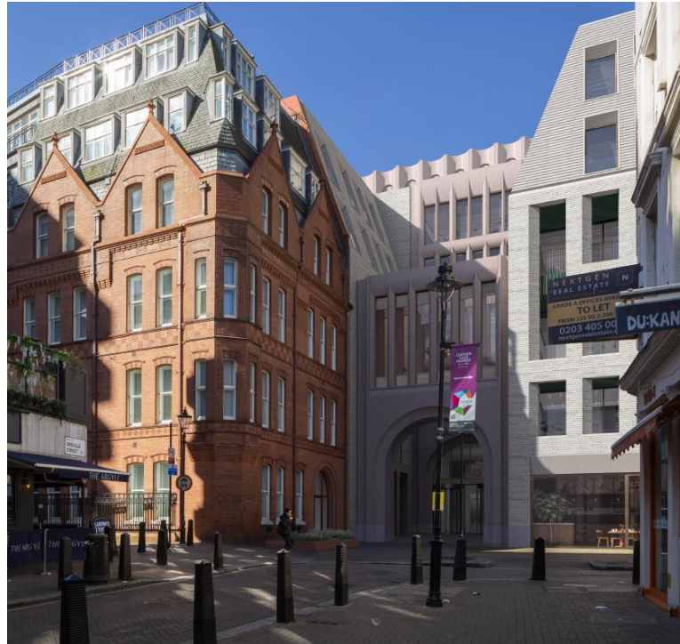
Figure 22. Image (right) shows new arched entrance which forms a continuation of Greville Street
