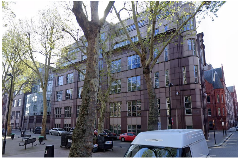
Figure 8. 1990s rear extension to 2 Waterhouse Square (from Brooke's Market).
