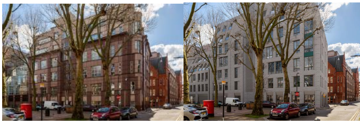
Figure 18. Before and after images of the existing rear extension and the proposed development, demonstrating the similar siting, scale and massing.
