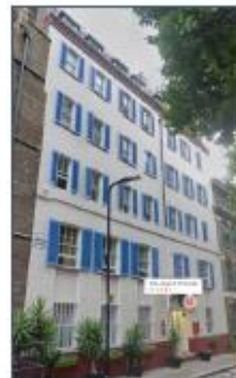
Figure 2: Street View of Front Elevation
