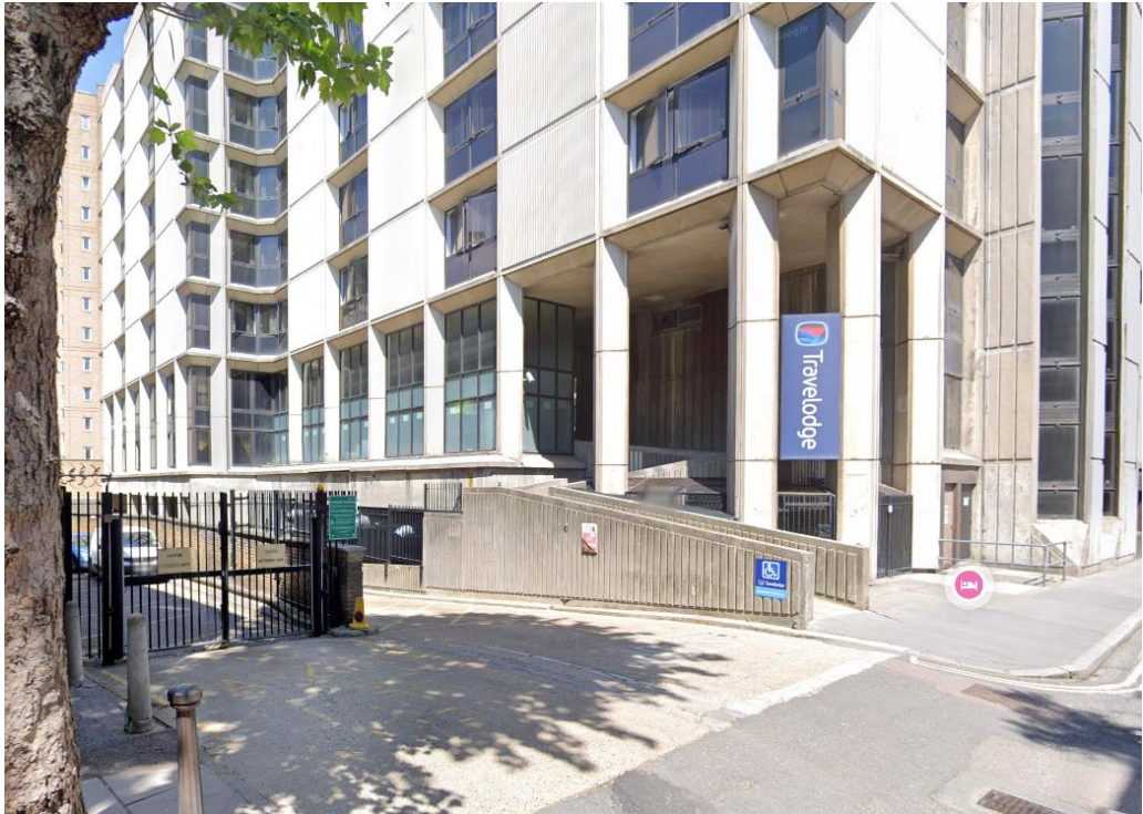
Figure 7 – View of existing rear elevation from Shorts Gardens
