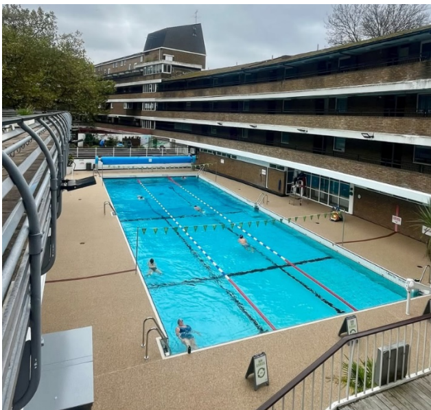
New Pool Deck at Oasis Sports Centre
