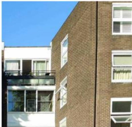
Windows in brick panels contrasting with light coloured panels with larger glazed areas.
