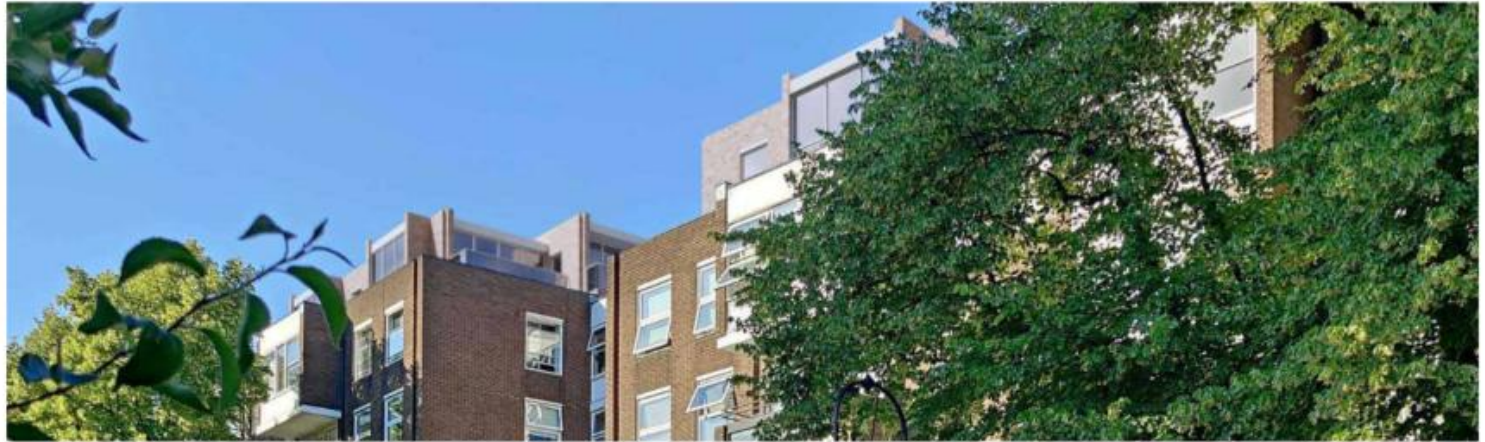
Proposed mix of windows in brick panels contrasting with light-coloured elements with larger glazed areas.
