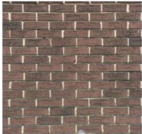
Close up of brickwork
