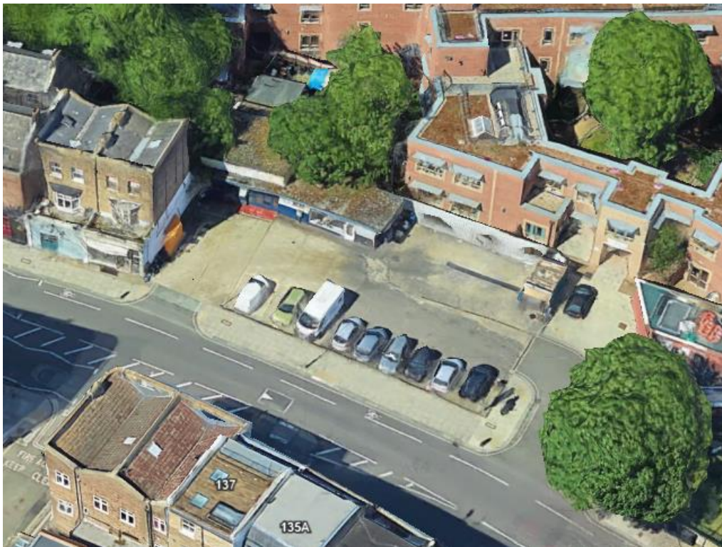
Figure 2 – The existing site (centre) viewed from the south
