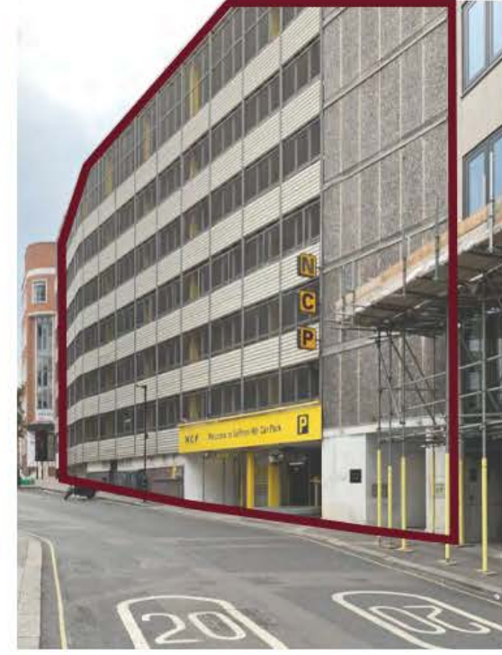
Car Park Entrance on St Cross Street, South Elevation
