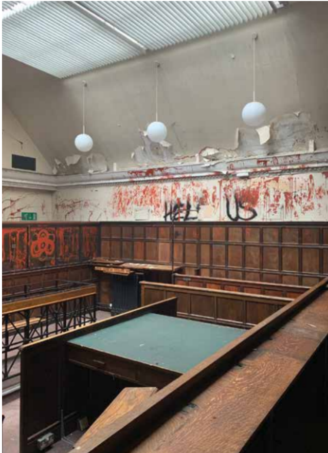
Photo 1: photo of court room
