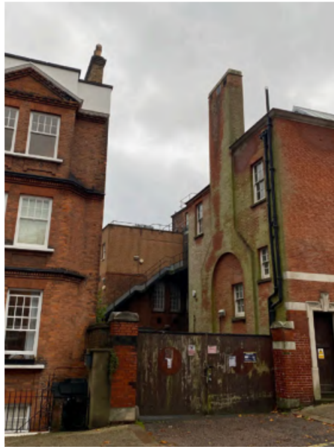
02. View from Downshire Hill
