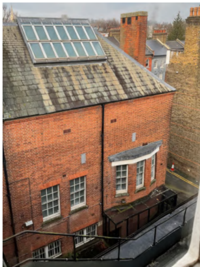
13. South Facade high level windows
