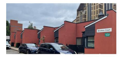
• **5-7 Belsize Grove** full retrofit which involved new windows, external / internal insulation, mechanical ventilation, solar panels and new more energy efficient radiators.
