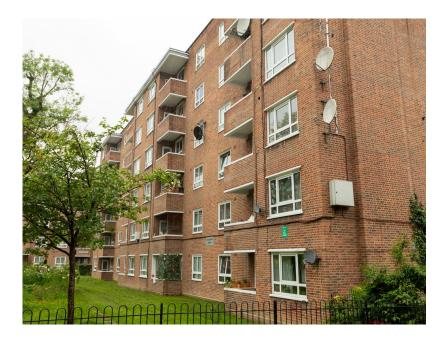
117-164 Kiln place – new flat roof system to the block with a 20-year warranty, new fire door sets to all properties in the block, new external fire retardant decorations, upgraded emergency and communal lighting, new windows with redesigned Juliet balconies to provide safer opening for families.
