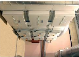
5k ESP and Three UV-C modules installed as an integrated system.
