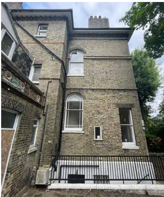
Figure 3. The windows on the flank wall to 10 Lyndhurst Road face onto The Cottage's front garden and existing roofscape. The Cottage's first floor is set back to accommodate one of these windows.
