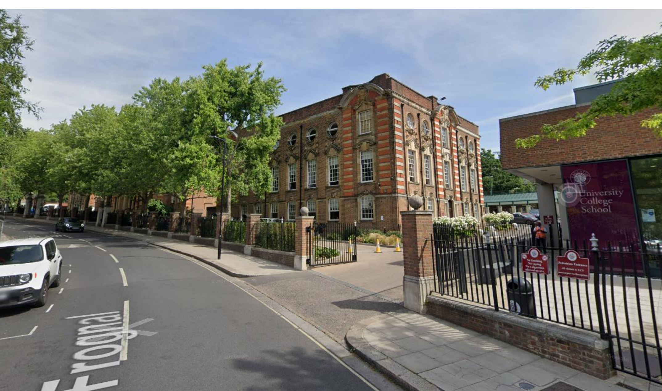
camden.gov.uk Street view from Frognaal showing listed front buildings
