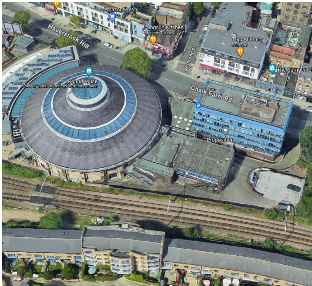
Figure 1 - The site viewed from the south
