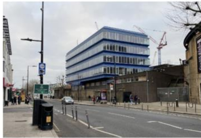
View of 100-100A Chalk Farm Road from north-west
