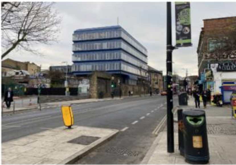
View of 100-100A Chalk Farm Road from south-east
