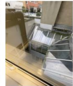
Roof of glazed 'link'
