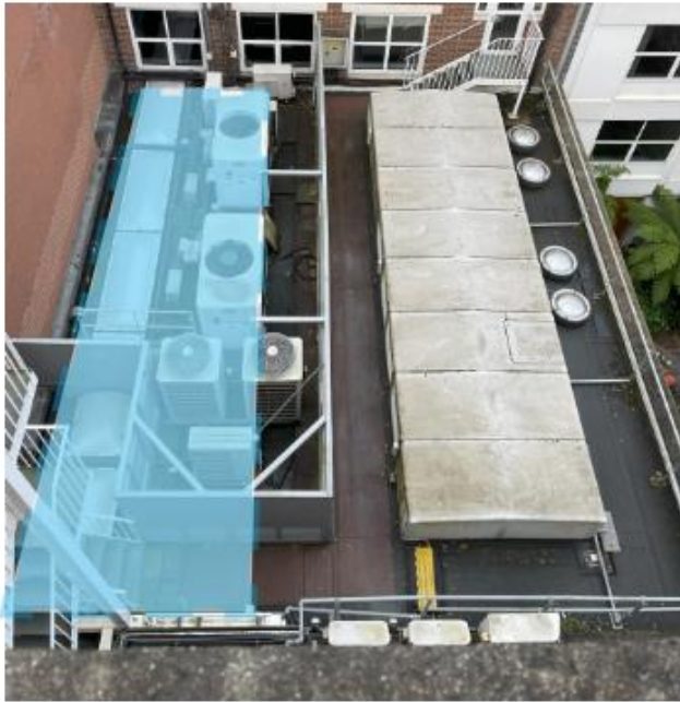
Existing Roof of 'Link' Structure
