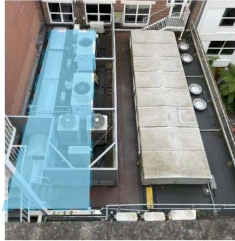
Existing Roof of 'Link' Structure
