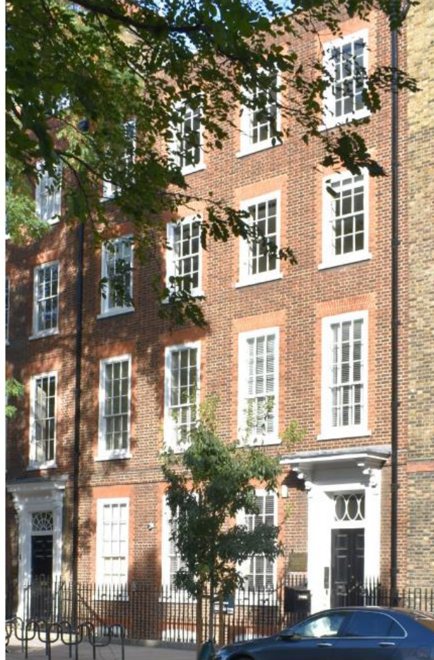
Rebuilt Elevation (Completed 1967)
