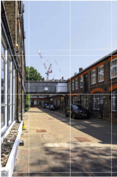
LINK BRIDGE - PHOTOGRAPH AS EXISTING
