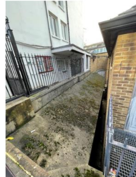
Above: Retaining structures to 36 College Crescent
