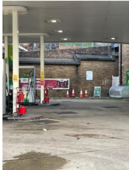
Above: Retaining structures support College Crescent
