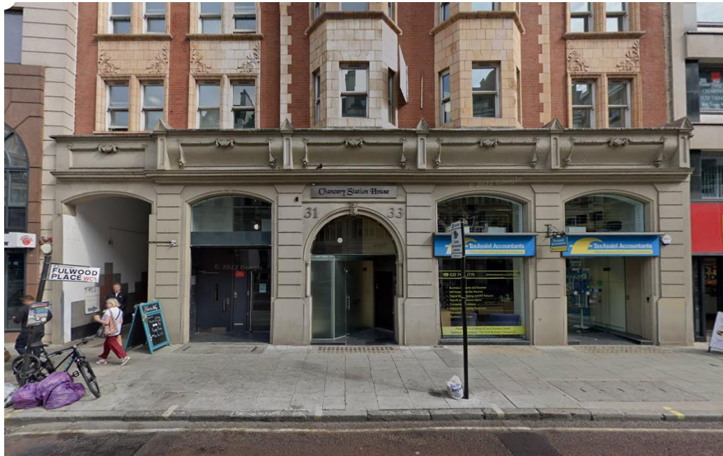
Figure 3: Existing front elevation of 31-33 High Holborn (Fulwood Place passage shown to left of frontage).
