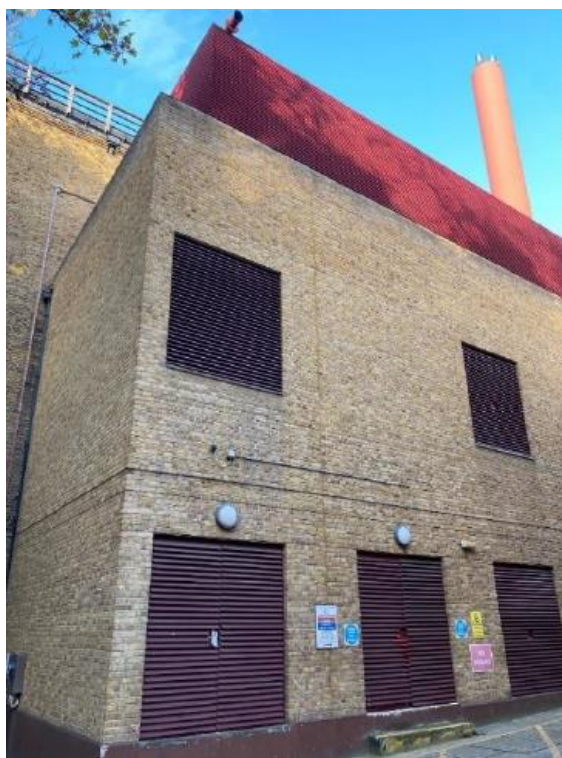
Figure 4 (above): Brick built South West Boiler House to be demolished
