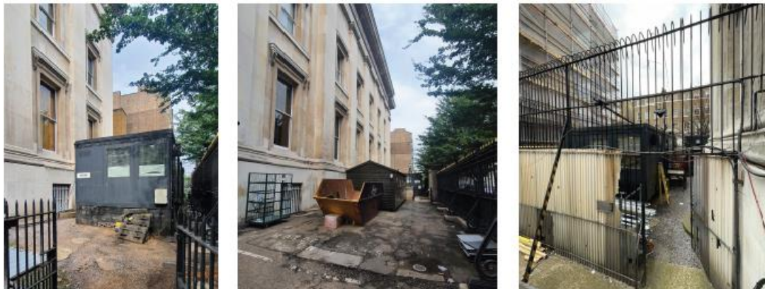
Figure 6 (above): South East portacabins to the north and east of the White Wing
