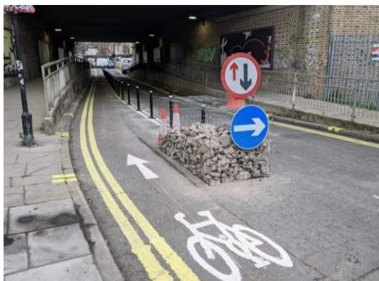
Figure 2: new northbound cycle lane underneath railway bridge, Camley Street
