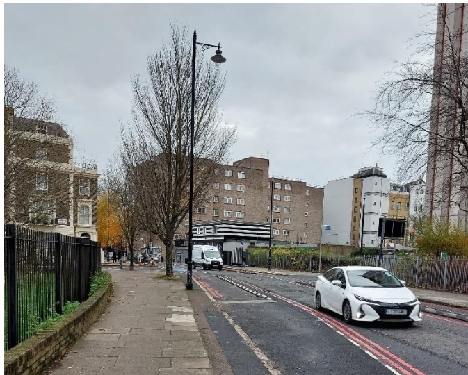
Figure 7: Harrington Square eastbound contraflow cycle lane on the TLRN
