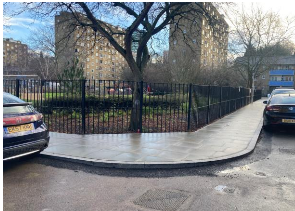
Figure 5: pavements replacing space previously reserved solely for parking, Cumberland Market
