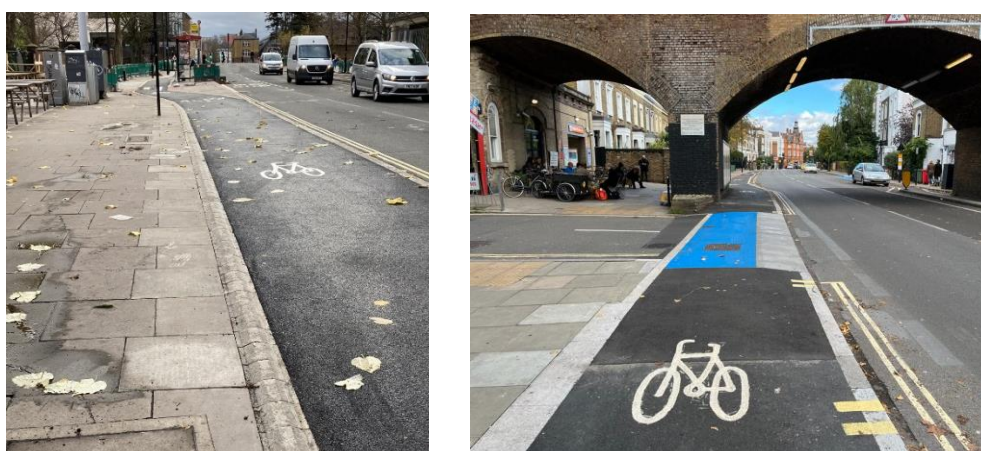
Figure 1: (left) York Way permanent scheme, (right) Prince of Wales Road final scheme
