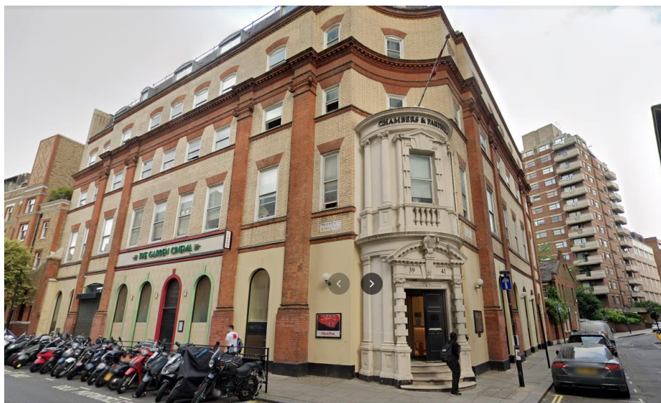
Figure 1 – The existing site
