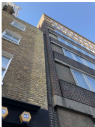
Contrasting scale between the existing building and Arthur Stanley House
