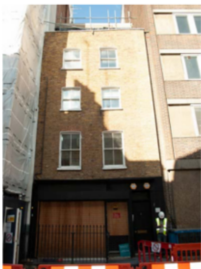
52 Tottenham Street front facade (basement lightwell has been infilled in recent history)
