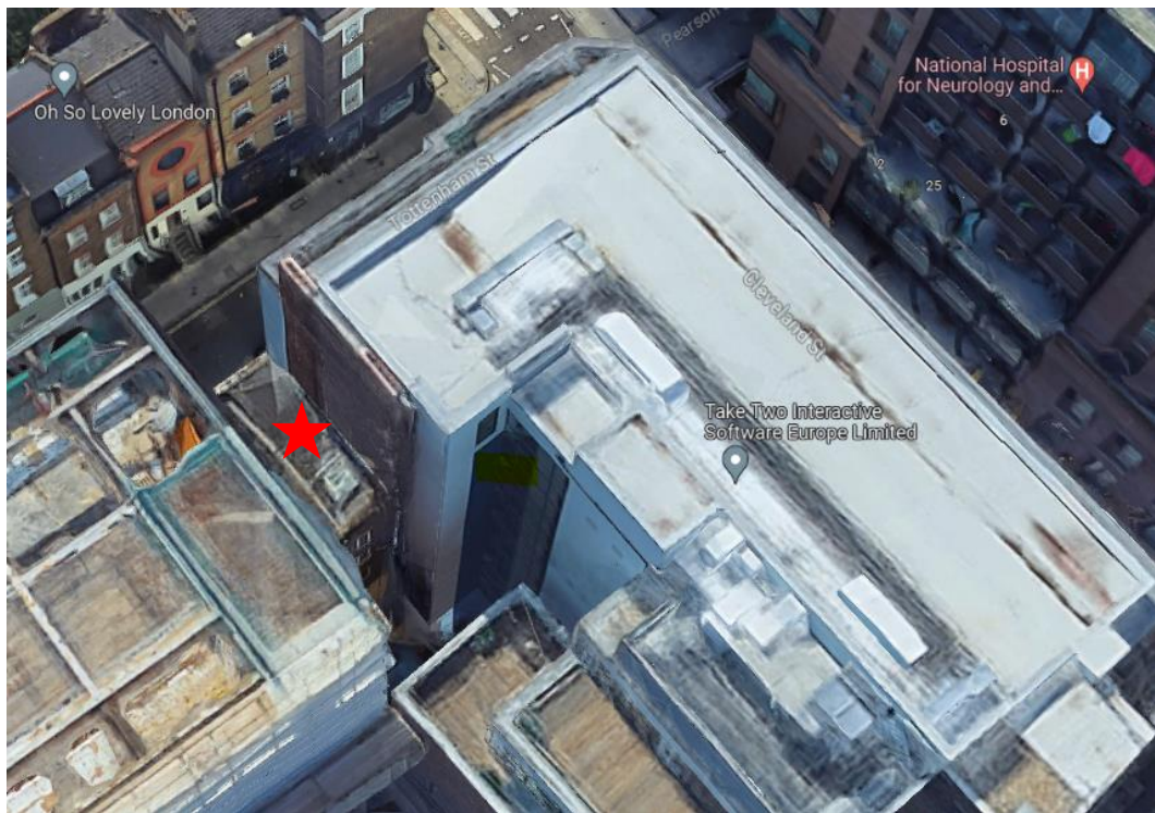
Figure 1: Aerial view showing the lightwell serving no.30
