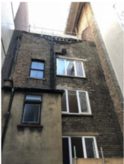
View of back elevation from above the ground floor extension.
