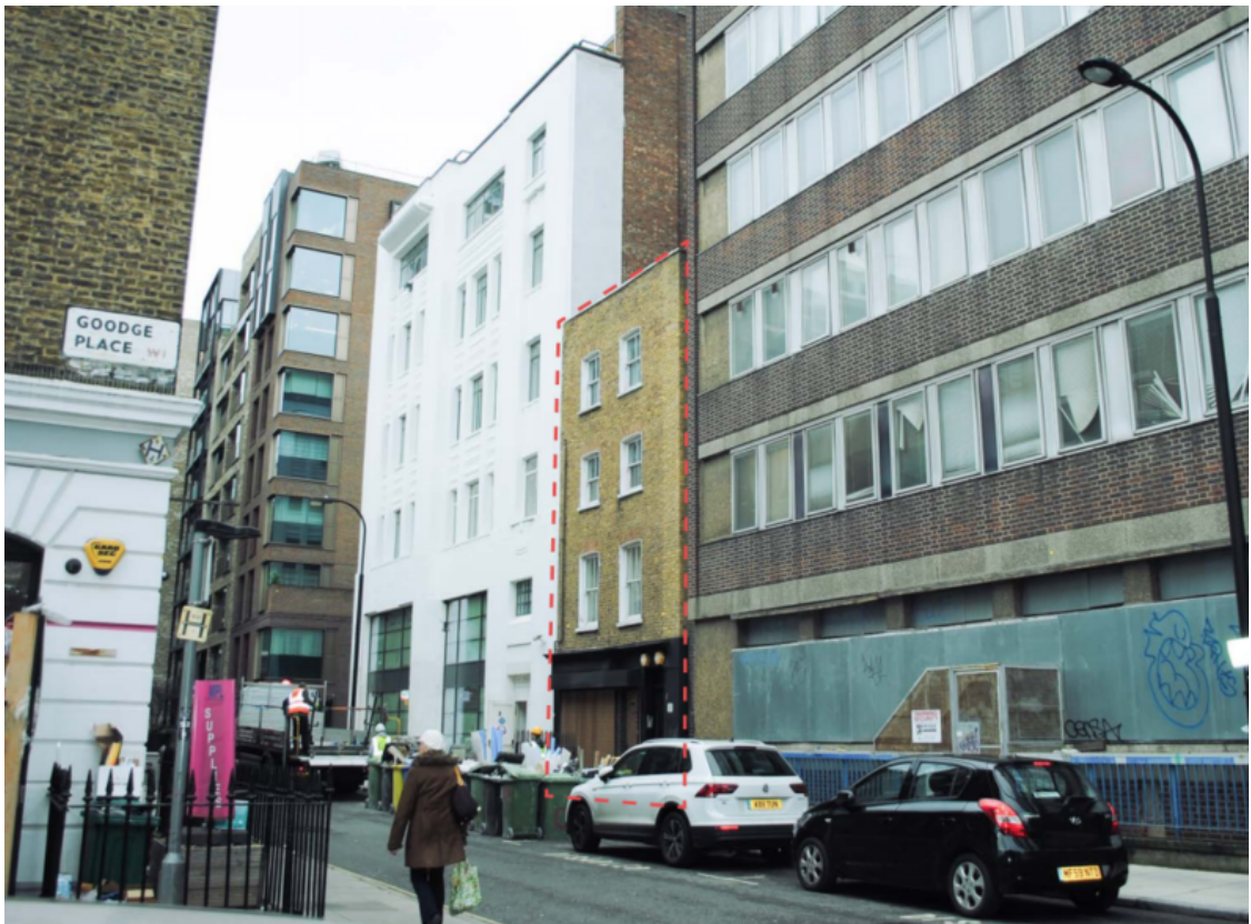
Figure 2: Street view of front elevation
