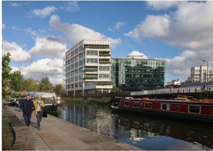
West and canal side elevations as seen from across Regent's Canal looking west
