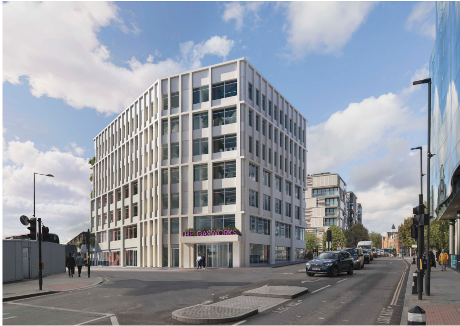
View of Building F1 from York Way looking north, with visible Goods Way, York Way and chamfered entrance frontages
