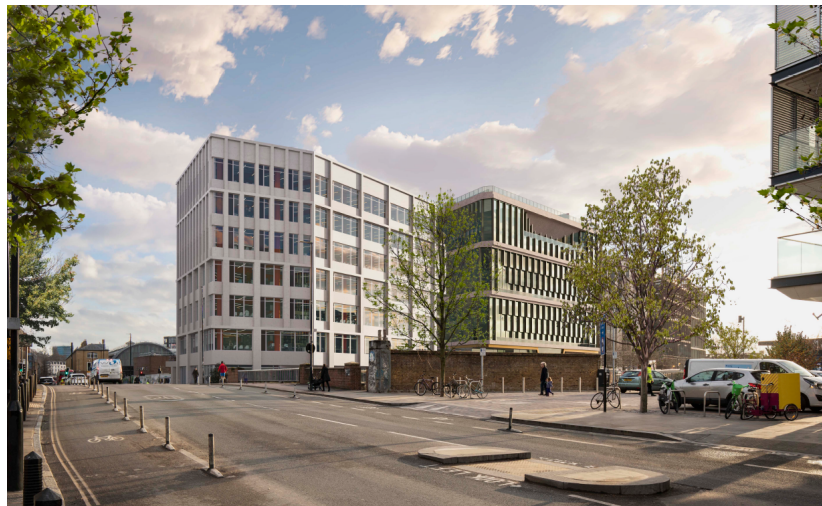
View of the canal side elevation from York Way looking south across the Maiden Lane Bridge
